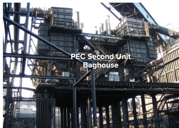
PEC Baghouse Infrastructure and PEC Baghouse Batteries 13–15 showing the coke guide enclosure, PEC hood and 13–15 & 19–20 PEC, or second unit, baghouse.
