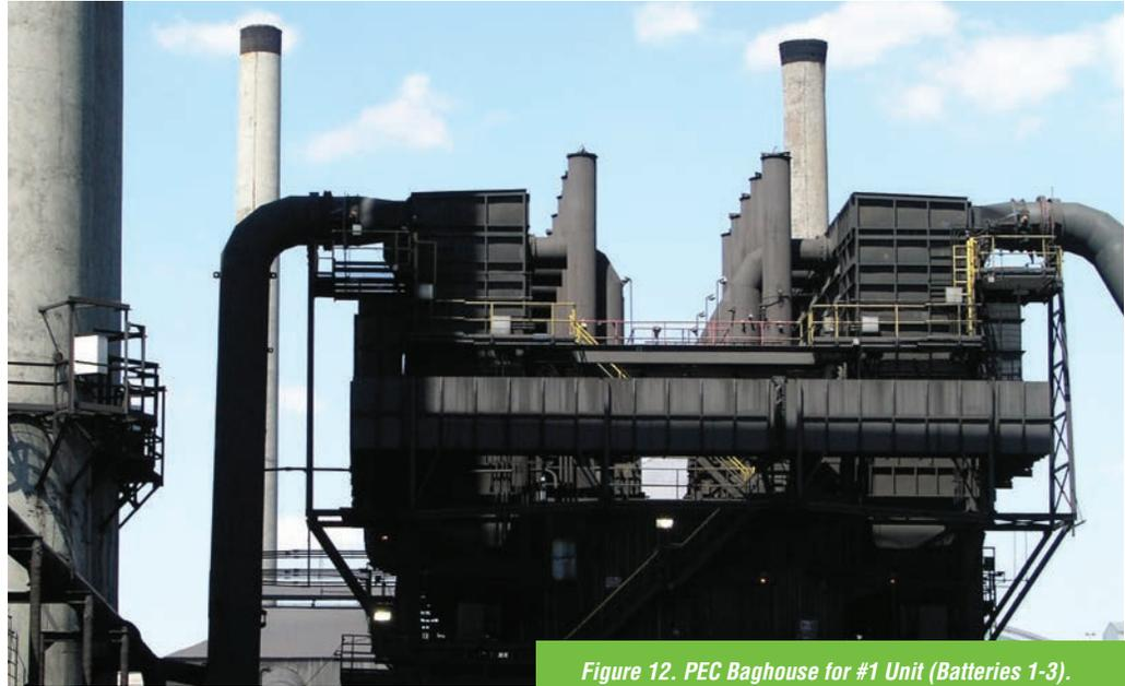
Figure 12. PEC Baghouse for #1 Unit (Batteries 1-3).
