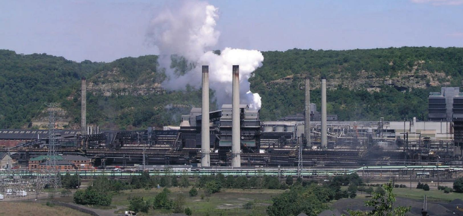
In addition to its superior efficiency and hydrogen sulfide removal, the state-of-the-art Clairton desulfurization process includes redundancy, which allows maintenance to be performed without losing the ability to desulfurize COG, whereas traditional by-product facilities require a two- to three-week maintenance outage at which time such facilities are not desulfurizing COG.
