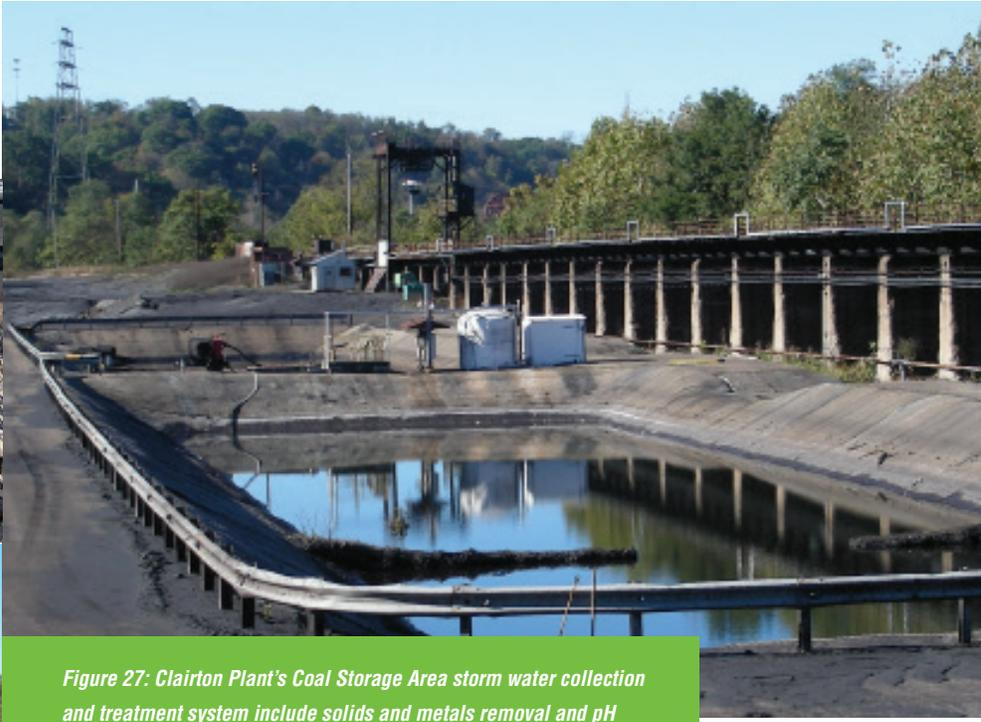
*Figure 27: Clairton Plant's Coal Storage Area storm water collection and treatment system include solids and metals removal and pH adjustment prior to discharge to the Monongahela River.*
