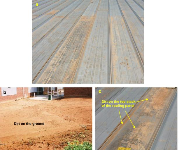
Figure 1. Photographs of stains and inconsistent appearance of a bare GALVALUME<sup>®</sup> roof (a), dirt on the ground at a building site (b), and dirt concentrated on the roofing panels on the top of the stack (c).
