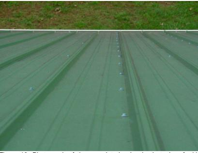
Figure 13. Photograph of the prepainted galvanized steel roof with non-matching screws.
