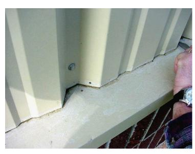
Figure 21. Photograph of premature corrosion on the bottom edge of the siding.
