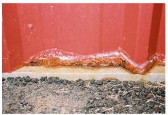
Figure 18. Premature corrosion at the bottom edges of the prepainted GALVALUME<sup>®</sup> panel caused by direct contact with the concrete foundation.
