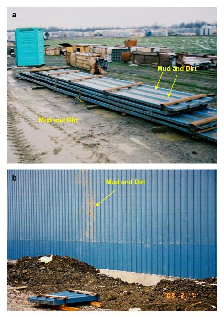
Figure 2. Photographs of mud and dirt on the prepainted GALVALUME<sup>®</sup> siding panels (a) before and (b) after the installation.
