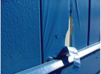
Figure 48. The topcoat delaminated from the primer.
