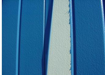
Figure 49. The primer remained on the panel where the topcoat peeled off.
