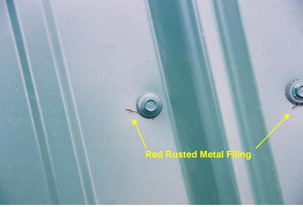
Figure 28. Photograph of red rusted metal filings from the screws on a prepainted GALVALUME<sup>®</sup> roof panel.
