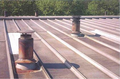
Figure 35. The GALVALUME<sup>®</sup> roof was corroded around the roof stacks.
