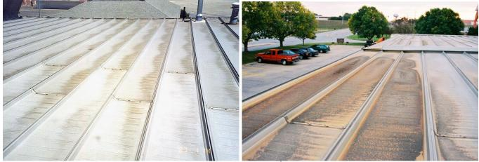
Figure 22. Photographs of water ponding on a GALVALUME<sup>®</sup> roofs due to improper slope of the roof.
