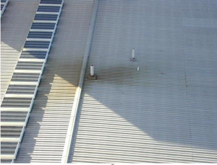
Figure 34. The bare GALVALUME<sup>®</sup> roof was corroded around the laboratory vent.
