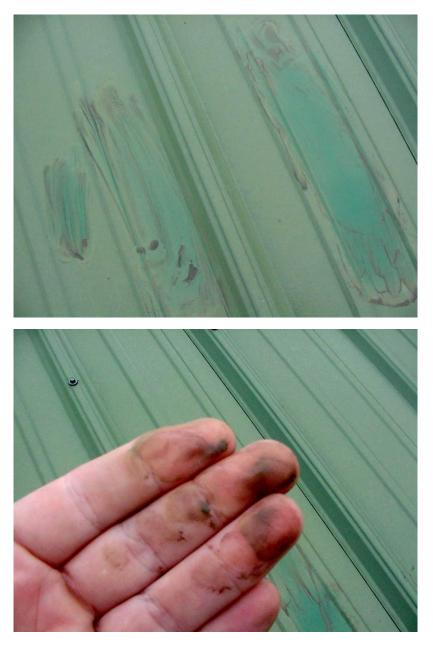
Figure 38. The prepainted GALVALUME<sup>®</sup> roof panel discoloration is due to dirt coverage.
