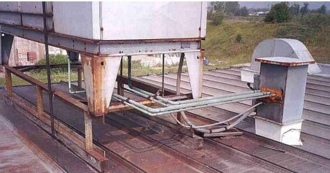
Figure 36. GALVALUME<sup>®</sup> roof panel corrosion due to condensation water runoff from the copper pipes.
