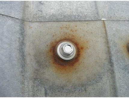
Figure 27. Photograph of red rusted metal filings on the surface of bare GALVALUME<sup>®</sup> roof panel around a screw.
