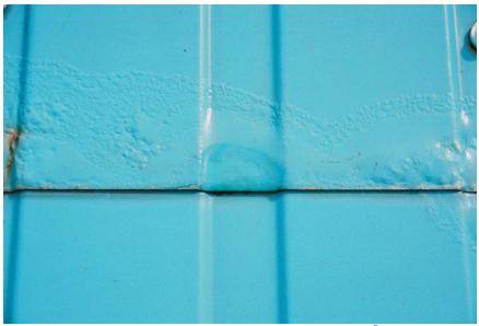
Figure 25. Paint blistering on a prepainted GALVALUME<sup>®</sup> roof caused by poor end lap sealing.
