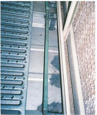
Figure 37. GALVALUME<sup>®</sup> panel corrosion due to condensation water runoff from the copper pipes.
