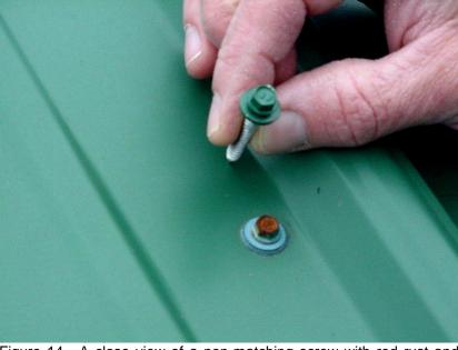
Figure 14. A close view of a non-matching screw with red rust and the correct screw, held in the hand, which should have been used for this application.
