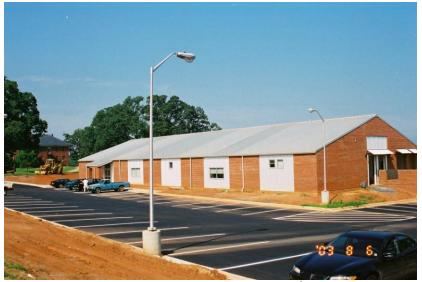
Figure 40. Differential darkening of ACRYLUME<sup>®</sup> panels on a high-slope roofing application.
