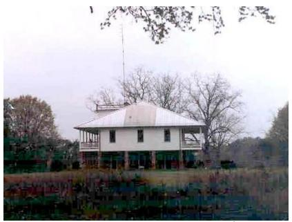
Figure 39. Differential darkening of bare GALVALUME<sup>®</sup> panels on a high slope roofing application.
