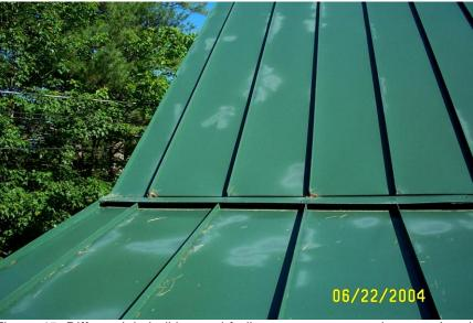
Figure 45. Differential chalking and fading appearance on the prepainted GALVALUME<sup>®</sup> steel roof with improper touch-up paint.
