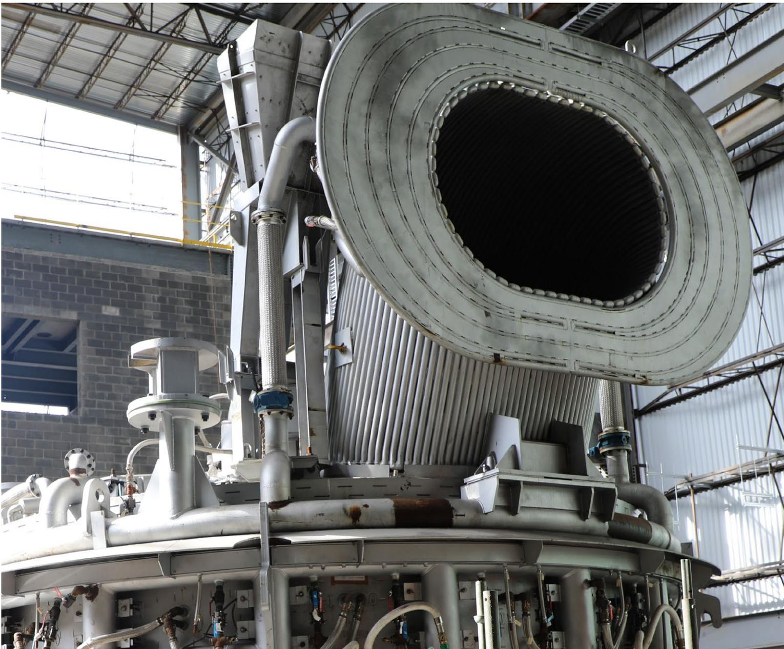
In the second half of 2020, we expect to begin operating a new state-of-the-art electric arc furnace (EAF) currently under construction at our Fairfield Works in Alabama, to produce several grades of tubular steel. These steels will be cast into blooms, also known as rounds, and subsequently pierced and heat treated at the facility's tubular finishing operations.
