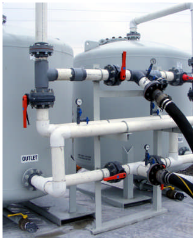
Granulated Activated Carbon (GAC) Vessels during the 2010 Pilot Study
