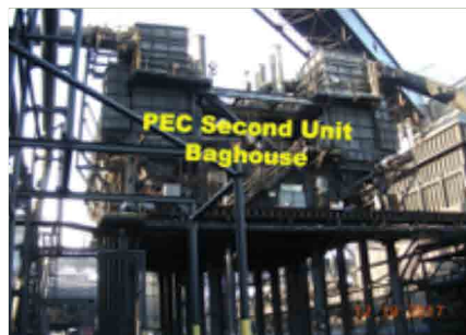
Figure 13. PEC Baghouse Infrastructure and PEC Baghouse Batteries 13-15 showing the coke guide enclosure, PEC hood and 13-15 & 19-20 PEC, or second unit, baghouse.
