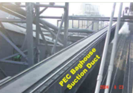
Figure 13. PEC Baghouse Infrastructure and PEC Baghouse Batteries 13-15 showing the coke guide enclosure, PEC hood and 13-15 & 19-20 PEC, or second unit, baghouse.
