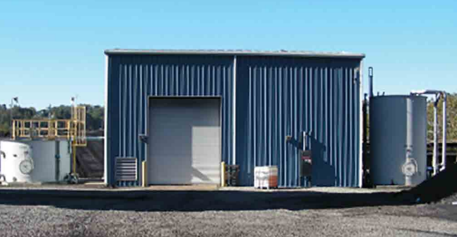
Figure 28: Clairton Plant's Coal Storage Area storm water collection and treatment system include solids and metals removal and pH adjustment prior to discharge to the Monongahela River.
