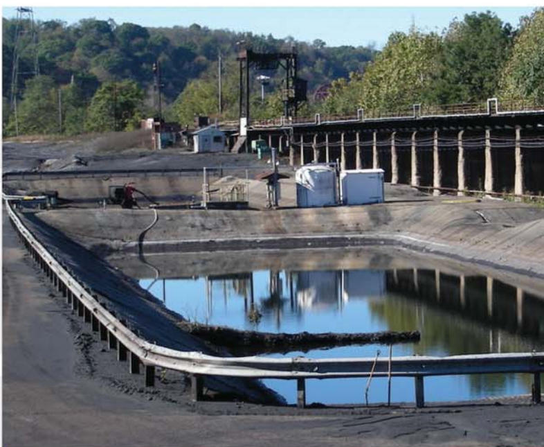
Figure 29. Clairton Plant's Coal Storage Area storm water collection and treatment system include solids and metals removal and pH adjustment prior to discharge to the Monongahela River.
