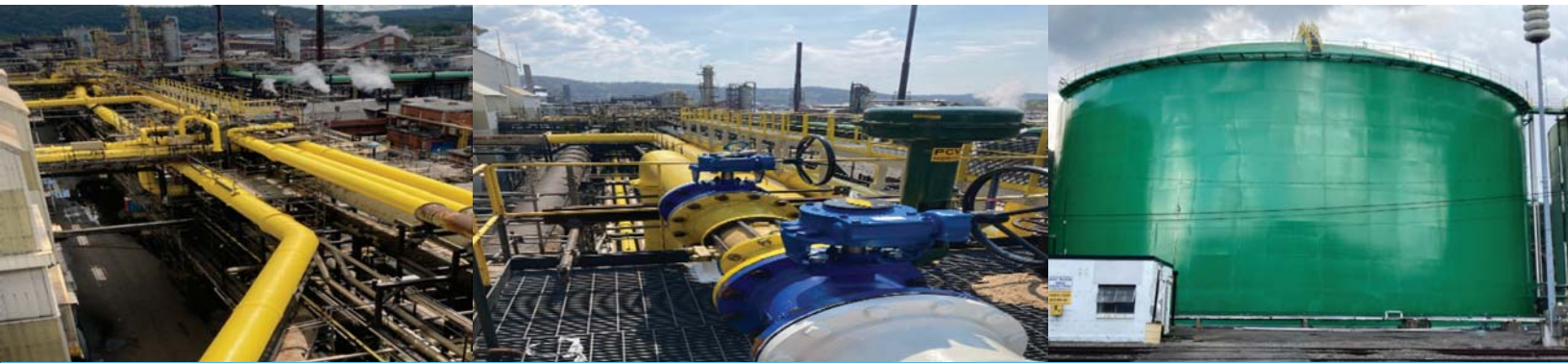
Figure 18. By-Products Piping and Tank Improvements.
