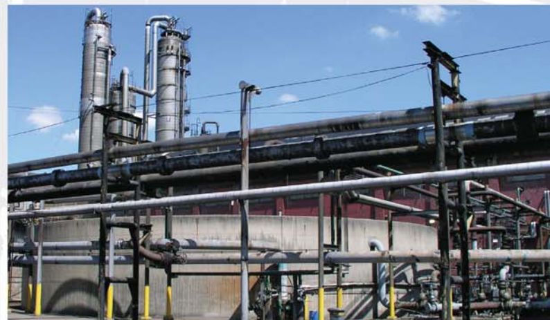
Figure XX. Biological Plant Ammonia Stills and Clarifier.
