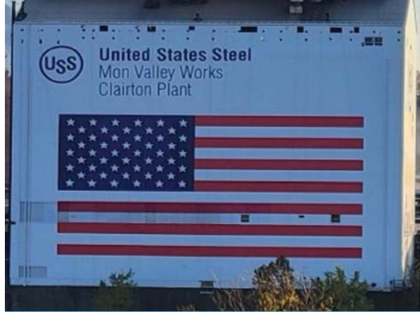
Figure XX. 2021 Boiler House Painting
